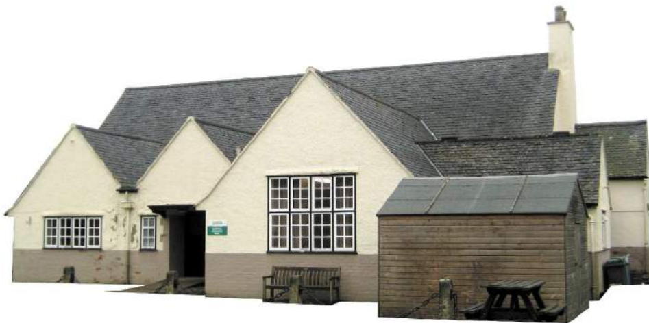
View of the hall as existing
